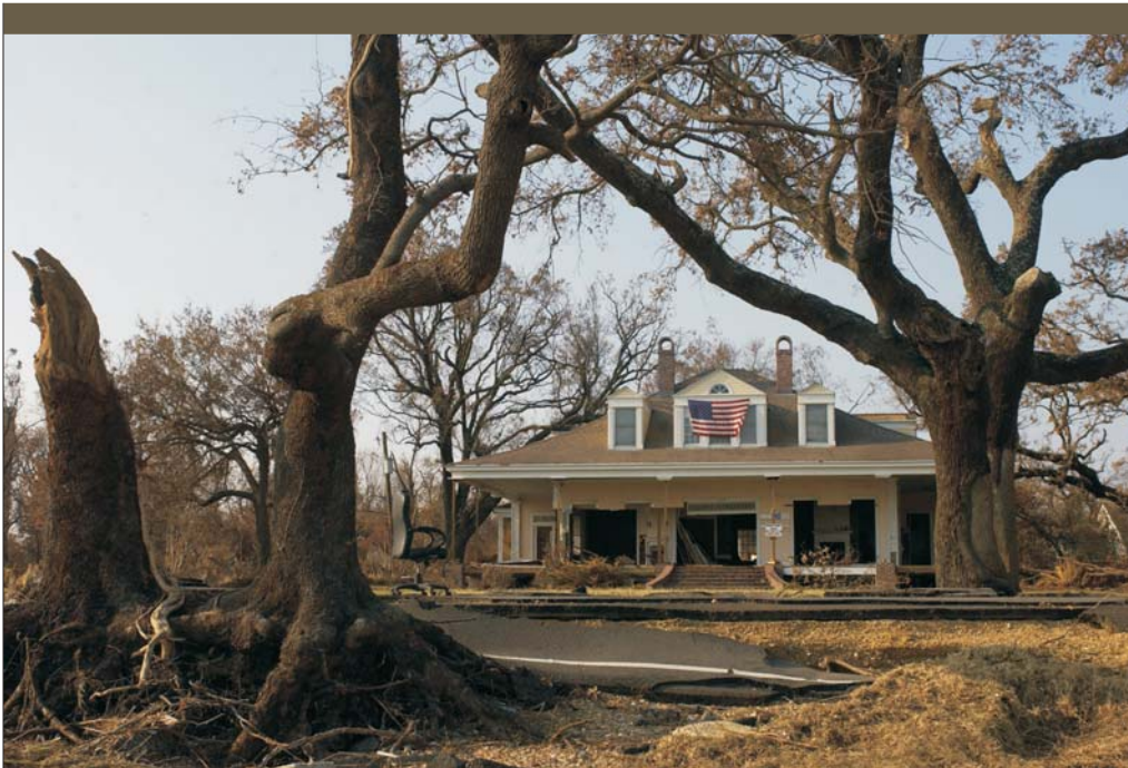
Storm destruction in Gulfport, MI. U.S. Air Force photo.
