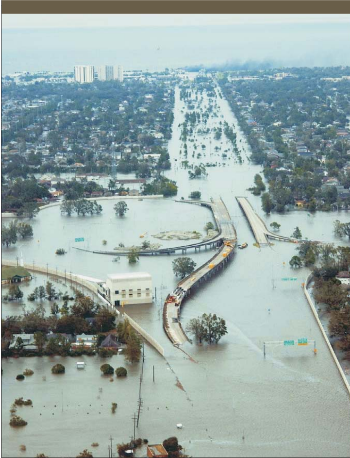
Flooded roadways of New Orleans. U.S. Coast Guard photo by Petty Officer 2nd Class Kyle Niemi.
