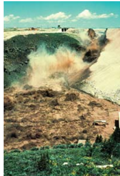
The Teton Dam in southeastern Idaho collapsed on first filling on June 5, 1976, causing the deaths of 11 people and $2 billion in damages.
